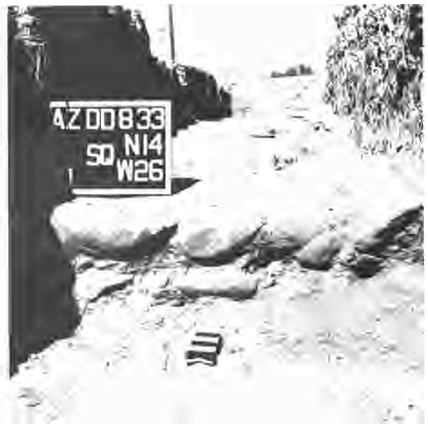
Figure 6. Cobble footing, south wall Room 12.
