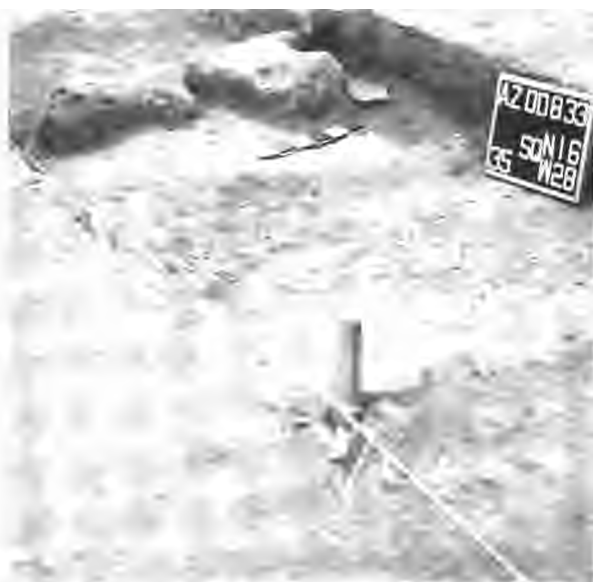
Figure 28. South wall, Room 12, in relation to upper adobe floor. Note wall fall on surface, at top.
