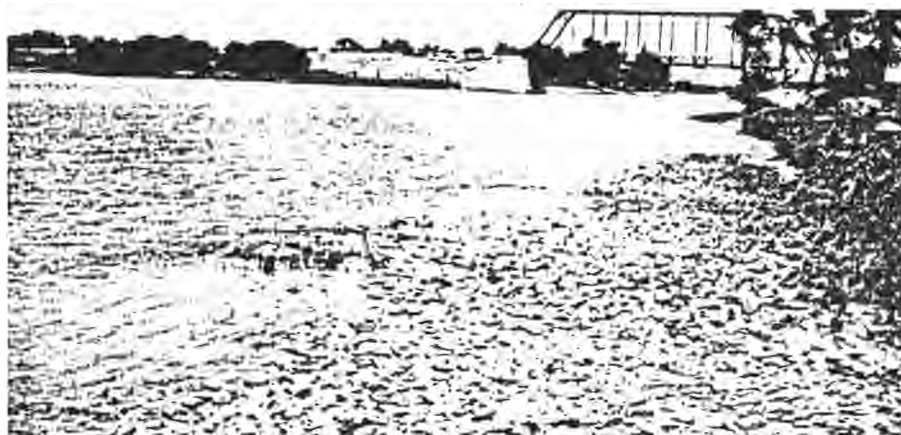
Station No. 2 Looking Upstream at the Little Colorado Bridge
