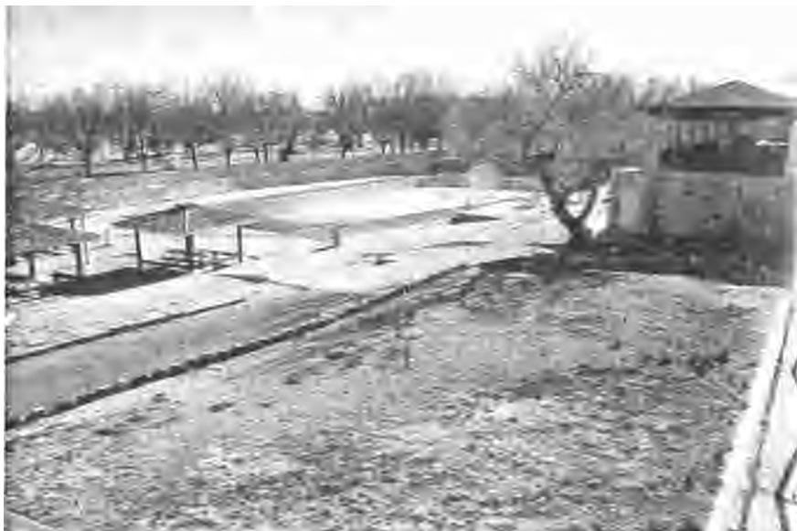
Figure 2.2. Comanche Springs was once at least the eighth-largest spring in Texas and has been a valued community resource since at least the 1500s by providing water for human utilization, habitat for aquatic organisms, and recreational opportunities. These were all lost when declining groundwater levels caused the spring to dry in 1961 (Brune 1981). The extinct source of the main Comanche Spring is present just in front of the building. (Photo by P. J. Unmack, 1996)
