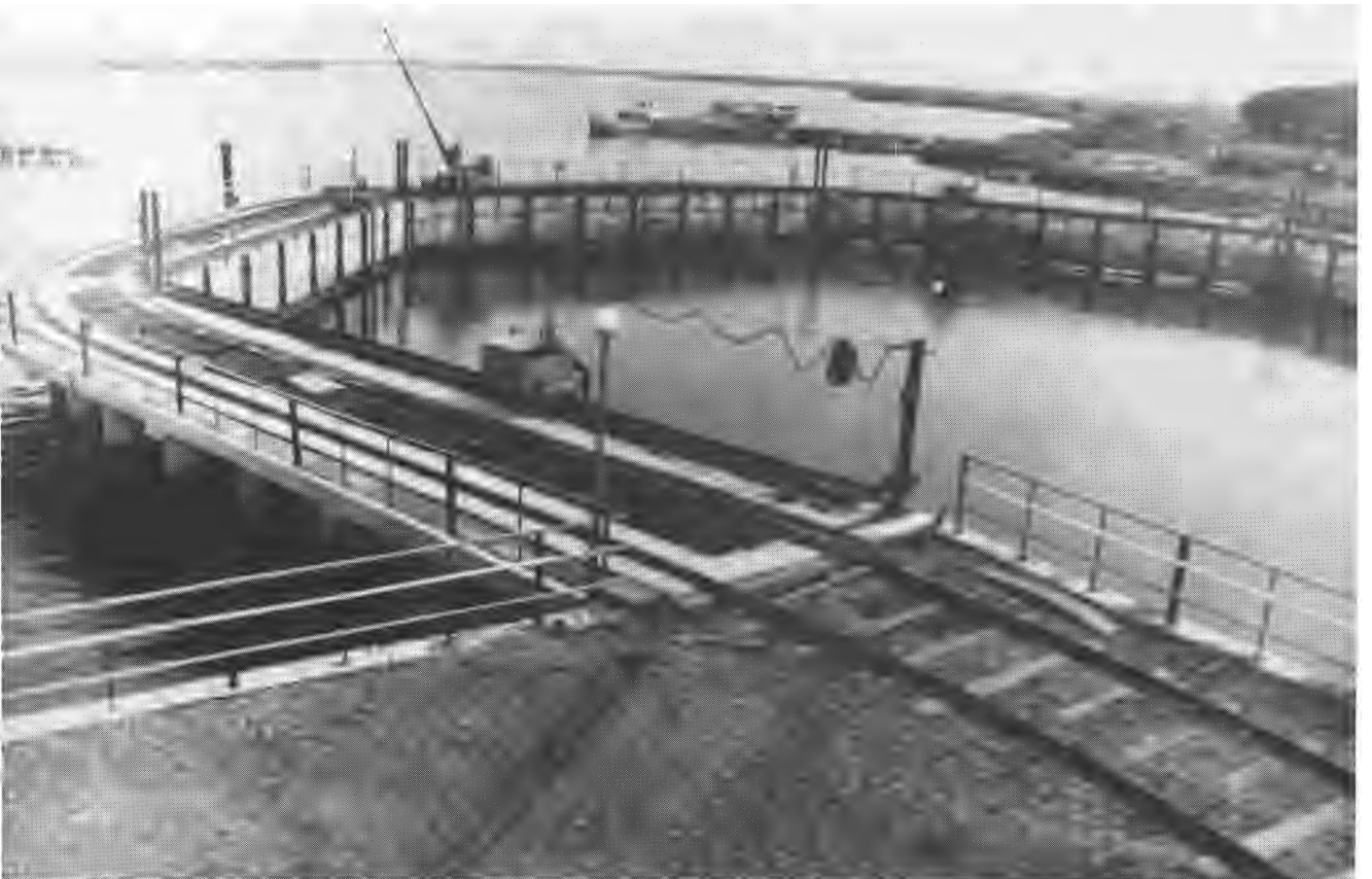
Plate 3. Fish protection screens with movable screen elements.
