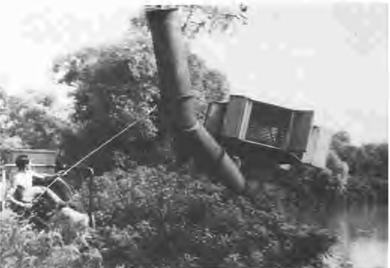
Plate 5. Placing the drum screen with blade at the water-intake head.
